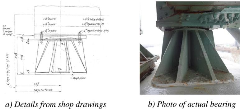
Figure 8. – Spherical bearings on Jacques-Cartier bridge.
